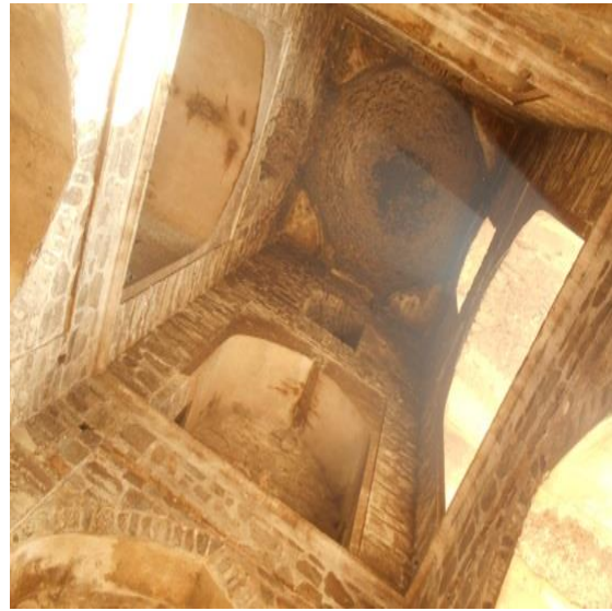
b. Roof covered with bats of Agrasen ki Baoli
