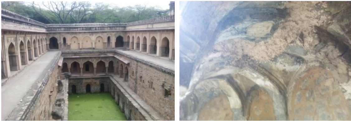
Figure 7 – a. Water covered with algae at Rajon ki Baoli b. renovated roof at Rajon ki Baoli
